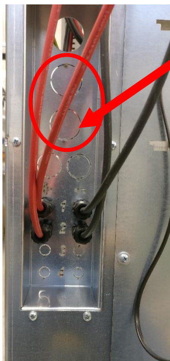
Picture 31 – Slots of Grid and EPS cables
