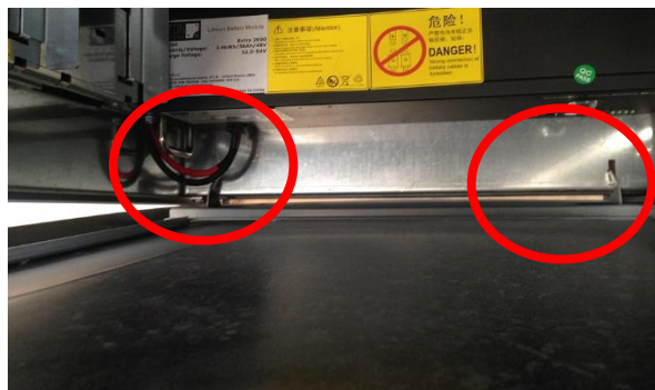
Picture 4 - Removal of the front panel
