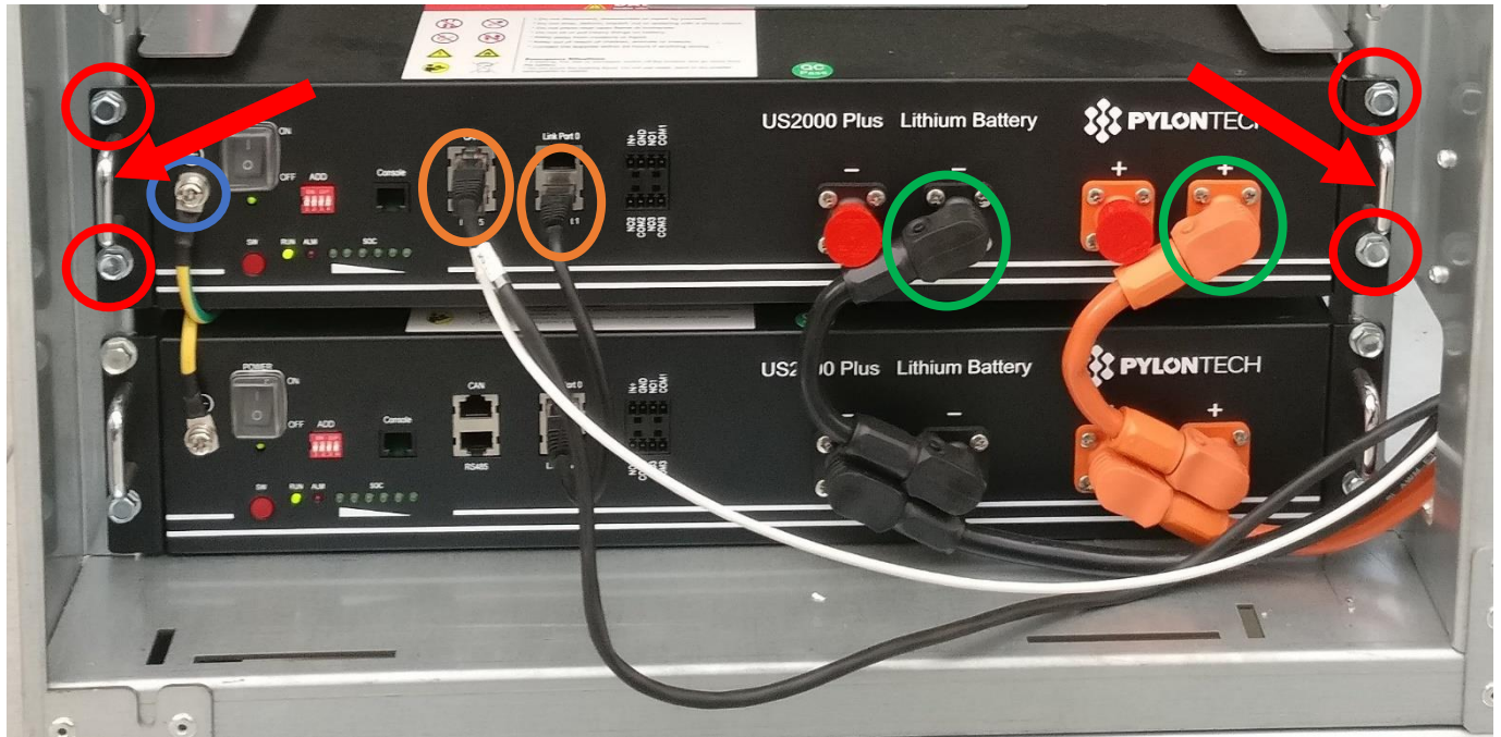
Picture 60 – Replacement of battery module – Removal module screws, equipotential bond screw, signal and power connections
