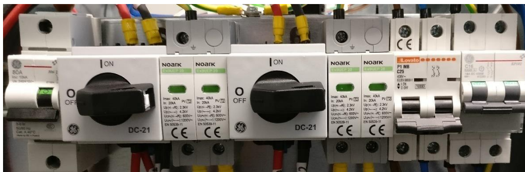
Picture 35 – Starting position of the protections of the RA.Store-K-F electrical panel
