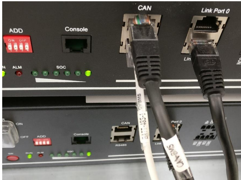
Picture 62 - Connection restore: data signals cables
