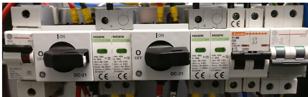
Picture 36 – All the breakers of the electrical panel in “ON” position
