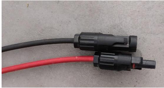
Picture 13A - Derivation cables from the string panel equipped with MC4 connectors
