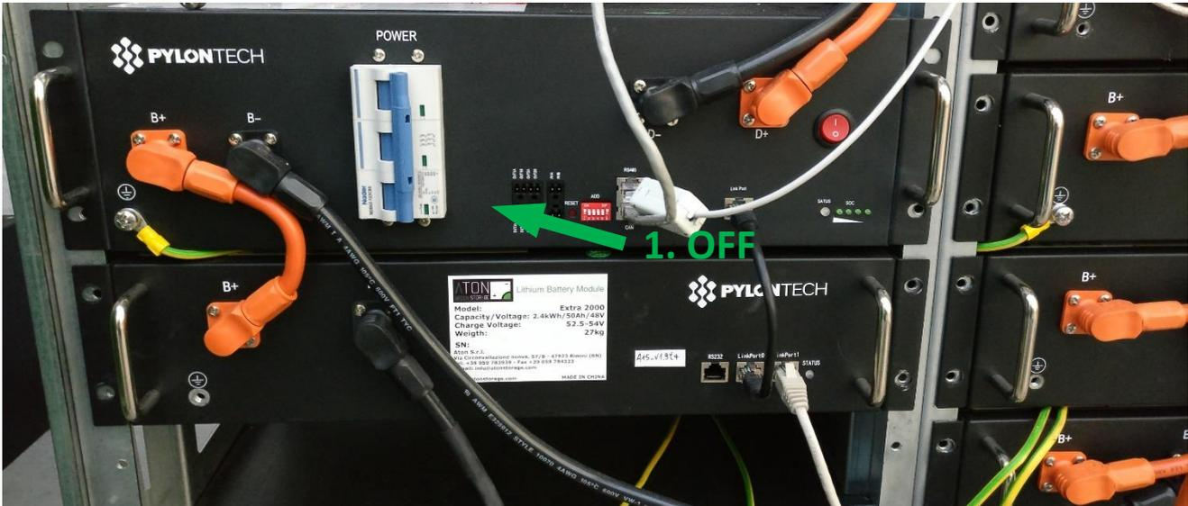
Picture B1 – Magnetothermal breaker of the batteries OFF (status indicator: green)
